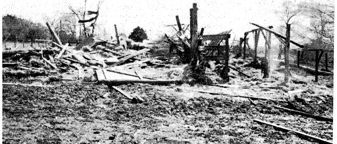
TORNADO DAMAGE — These photos reveal some of the damage done last Thursday morning by a tornado that touched down in Greenwood. Top photo shows the remains of a mobile home owned by O. C. Dunaway. The bottom photo, taken by Earl Collins, shows a pile of rubble that was once a dairy barn belonging to M. A. Schack.
